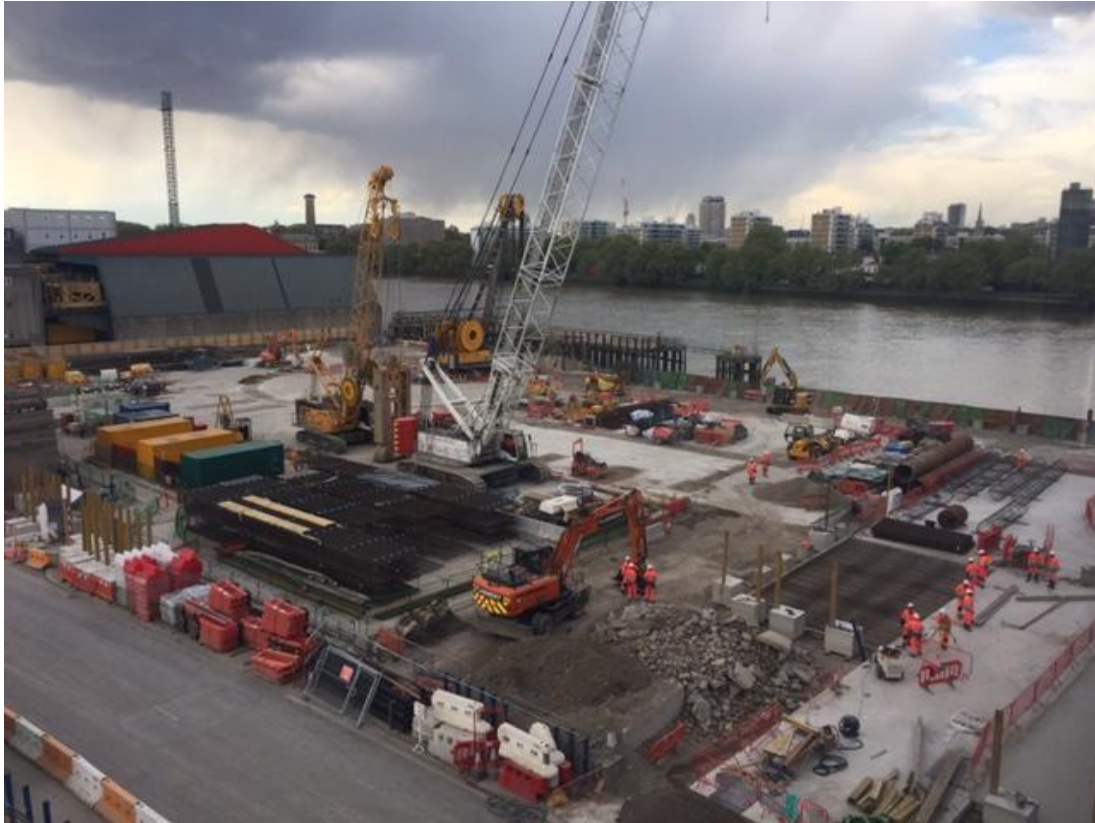
Figure 4: Construction underway: Kirkling Street double drive construction site (August 2017)
